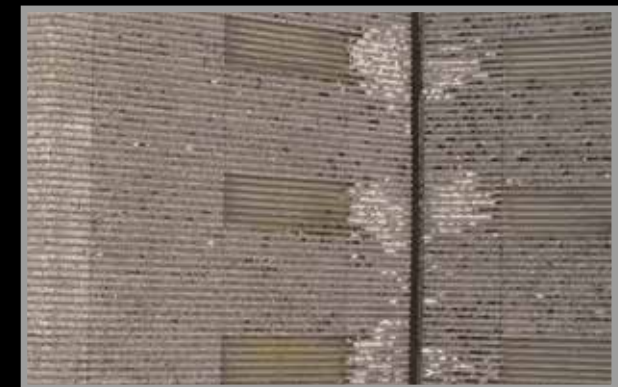
Delamination of panels – leading to structural degradation
